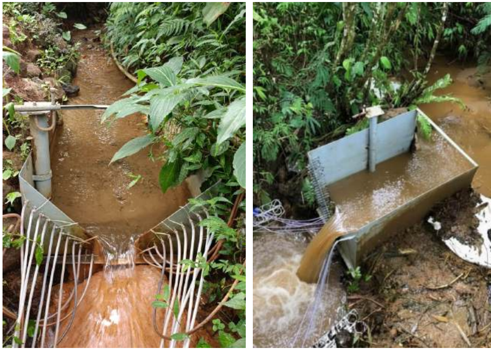
Figure 2 90° V-notch weir monitoring stations in the Leksana catchment (left) and Binangun catchment (right)
