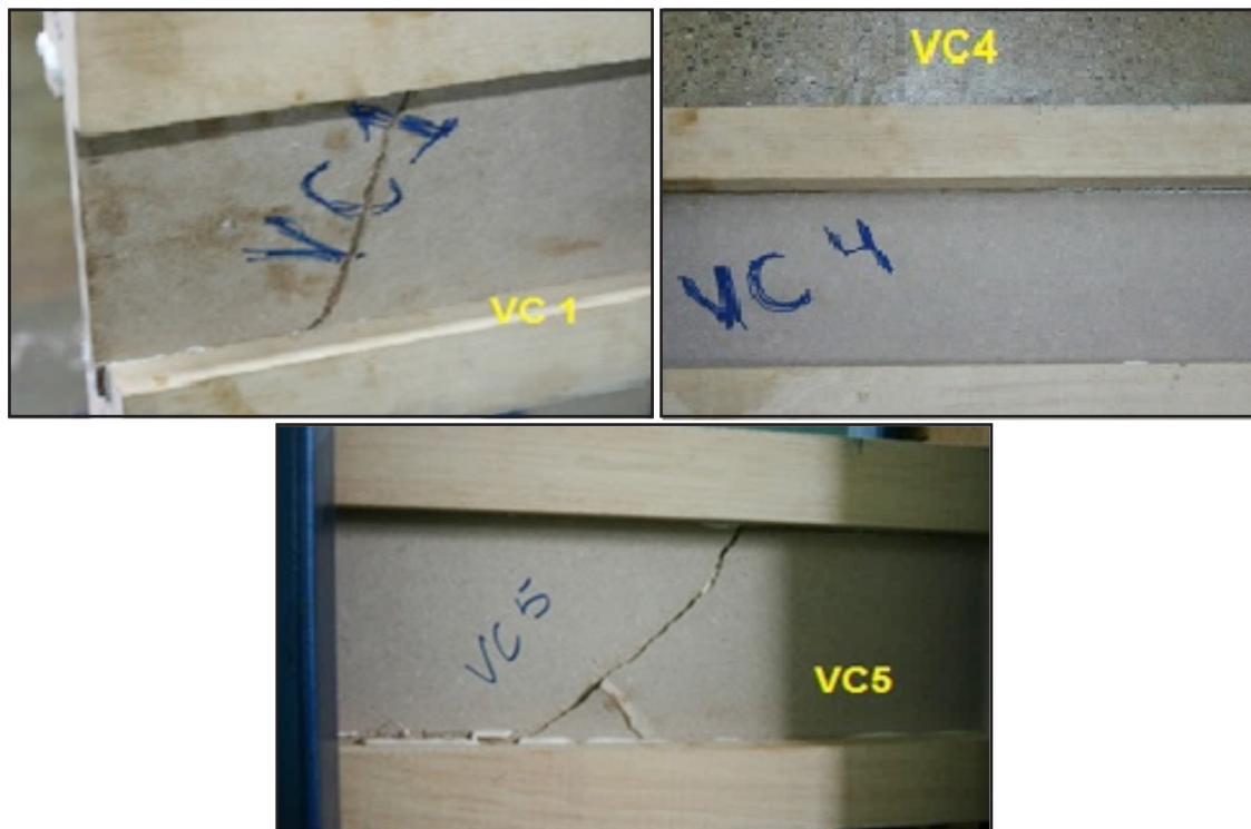
Figure 5 Rupture mode (ZW) observed for curupixá flanged wood I-joist
